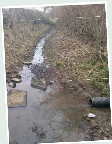
Thornley-with-Wheatley BW58 – Bridleway flooded by a pipe draining a field
