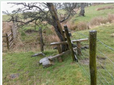
Newton-by-Bowland FP17 – Stile with loose steps and posts
